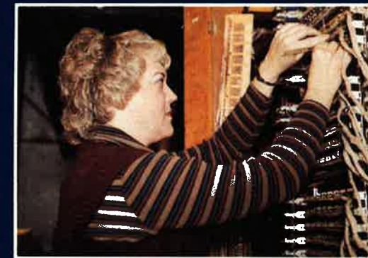
Sonia Carlson wires in new gang switches on the organ switch board.
