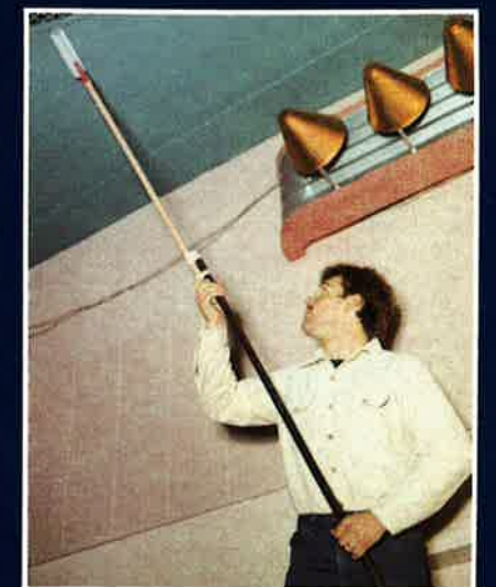
Jay Kleinjan gets ready to paint balcony ceiling.
